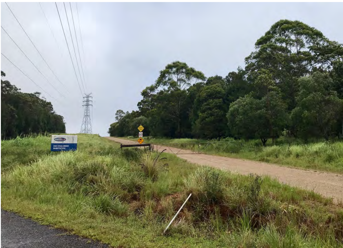
Entry to Chalumbin Substation Wooroora Station, off Tully Falls Road
